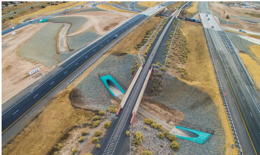
I-25 and NM-14 Cerillos Road in Santa Fe. Photo: Molzen Corbin.
