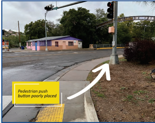
Figure 3: Intersection of NM 90 and Broadway Street
