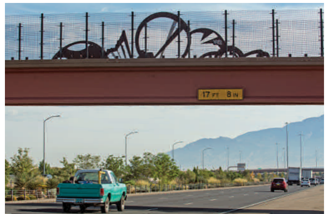
Figure 22. I-40 at Unser Boulevard.
