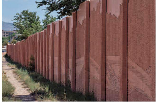
Figure 30. Noise wall along the Big I.
