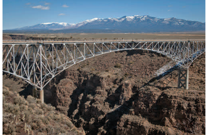
Figure 12. Rio Grande Gorge Bridge.
