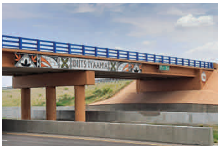
Figure 42. Exit 96 at McCartys. Note artistic design on girder and abutment; coloring on pier, abutment, and slope pavement; and texture on abutment.
