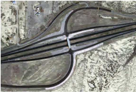
Figure 40. I-40 Exit 96 on Acoma Pueblo (image from Google Earth).
