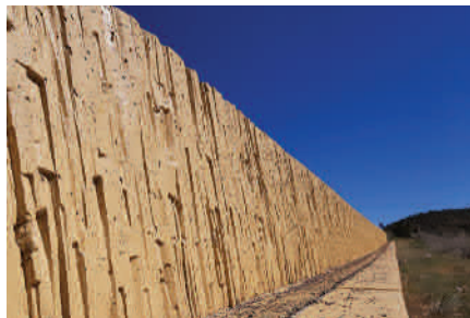
Figure 5. Cañoncito Interchange, I-25.
