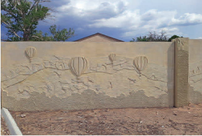
Figure 29. Noise Wall along NM 528 in Rio Rancho.
