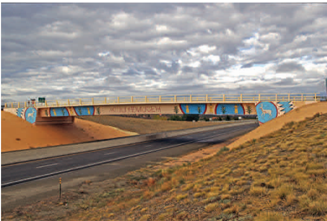
Figure 13. US 285 Overpass south of the Buffalo Thunder Resort Exit.
