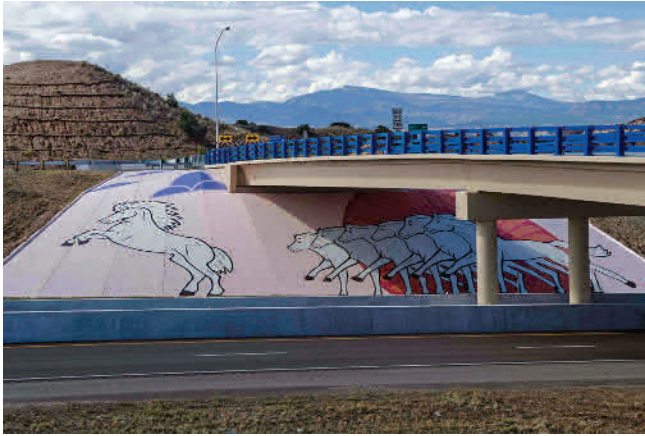
Figure 19. US 285/Arroyo Seco Interchange.
