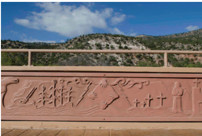
Figure 21. NM 4 at Jemez Springs.
