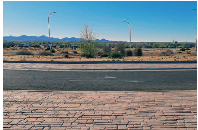
Figure 39. Stamped concrete lines the inner and outer portions of the roundabouts. The inner portion is contoured to collect rainwater and is landscaped with native vegetation.
