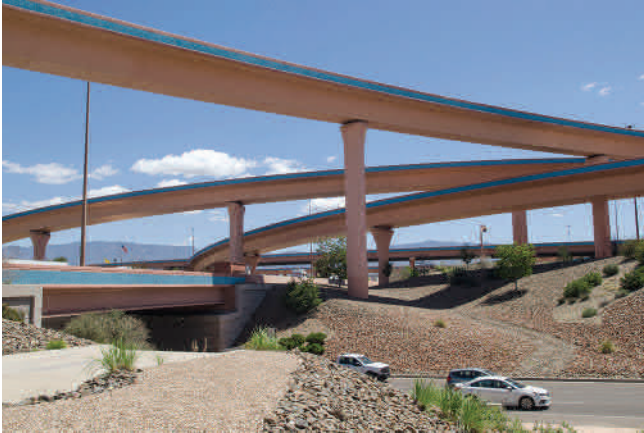
Figure 11. Big I Bridge Structures.
