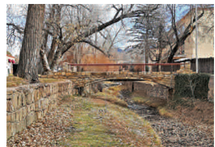
Figure 1. Civilian Conservation Corps-constructed stonework, Santa Fe River Park, Santa Fe.
