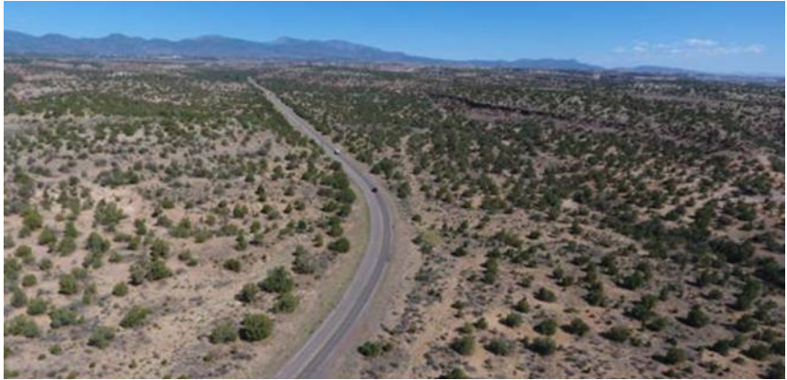
Tight Curve located North of Rover Blvd.
