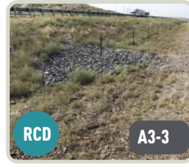
RCD A3-3 ROCK CHECK DAM
