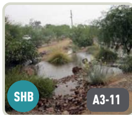
SHB A3-11 STORMWATER HARVESTING BASIN
