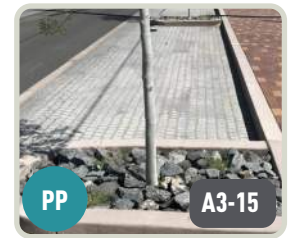
PP A3-15 PERMEABLE/ALTERNATIVE PAVEMENT
