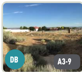
DB A3-9 DETENTION BASIN
