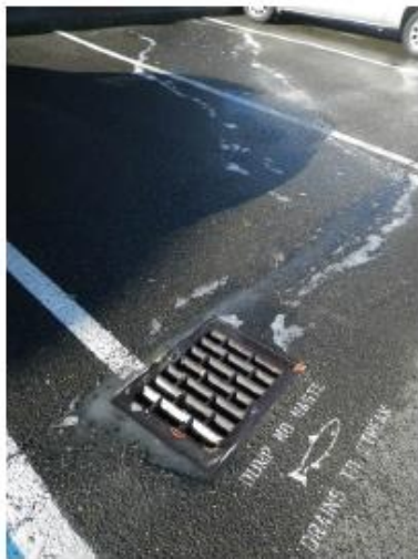
Wash water draining to a storm drain (photo courtesy WSDOT)
