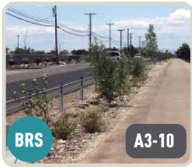
BRS A3-10 BIO(RETENTION) SWALE
