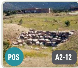
POS A2-12 POND OUTFALL STRUCTURE
