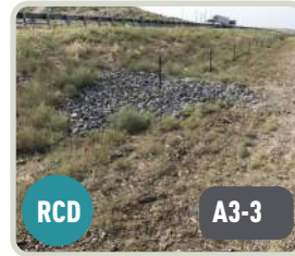
RCD A3-3 ROCK CHECK DAM
