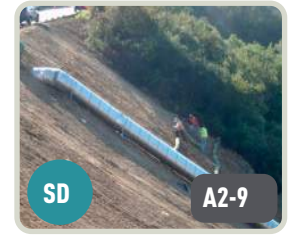
SD A2-9 SLOPE DRAIN
