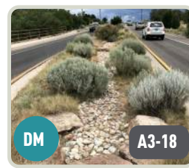
DM A3-18 DEPRESSED MEDIAN
