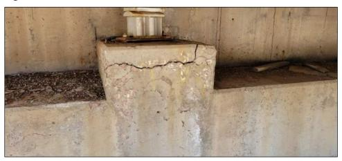
The columns have moderate vertical, horizontal, and map cracks (Figure 33), with isolated spalls and delamination at pier 2 column 3, with up to 2 in. of exposed rebar, and pier 1 column 3 has delamination. Pier 2 column 1 has a diagonal crack full width. Pier 1 column 3 has 8 in. of exposed rebar.
