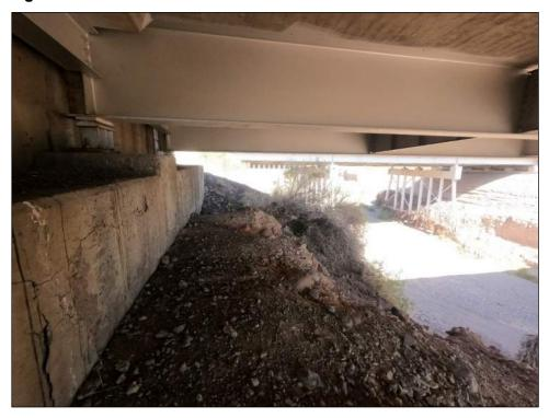
The pier caps have moderate vertical, longitudinal, and transverse cracks. Minor delamination and some evidence of repair with signs of patching are evident.
