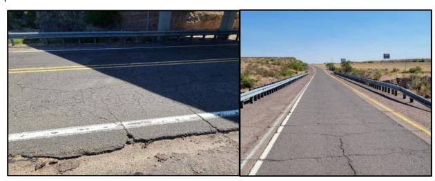
Figure 18: Pavement Condition on a Sample Ramp
