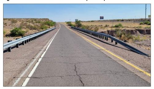
Figure 25. Pavement Condition on US 380 under I-25 Bridges
