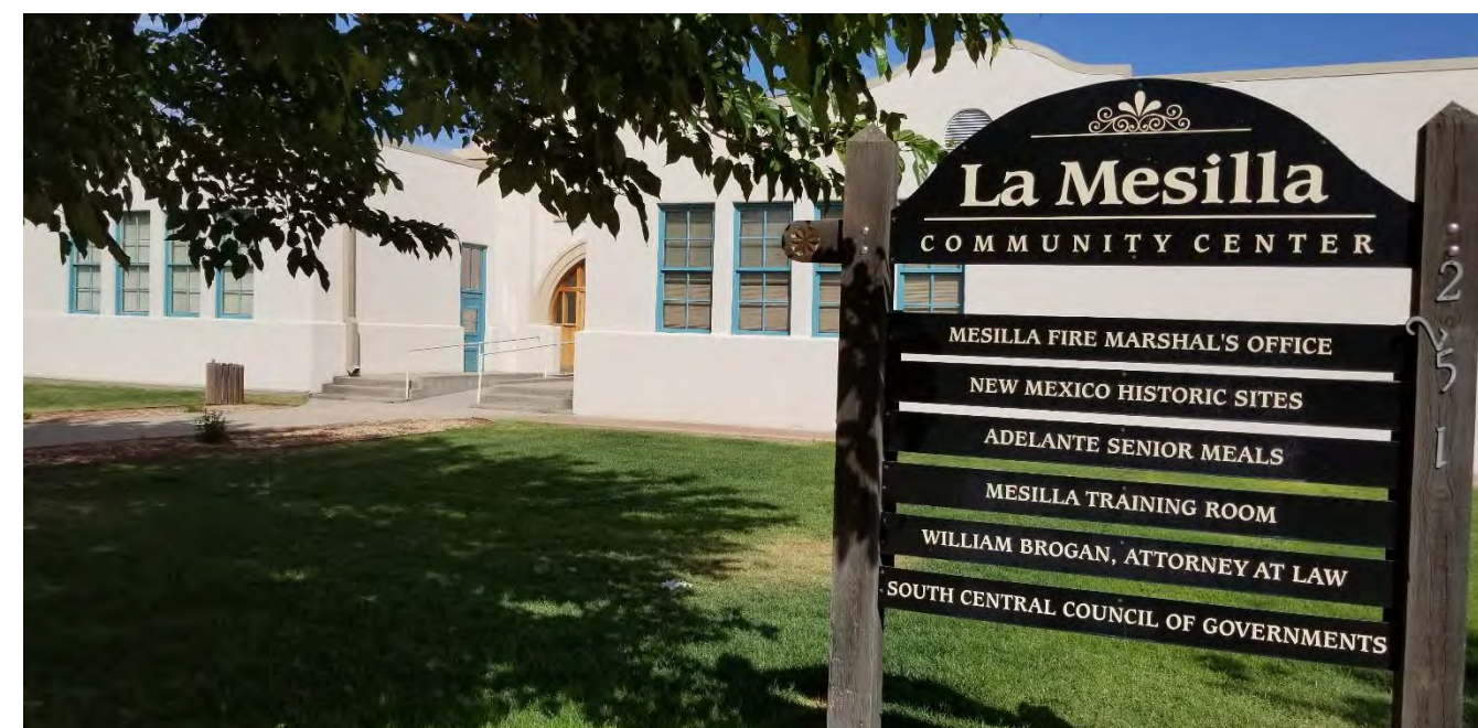
Figure 2.1.1 La Mesilla Community Center
