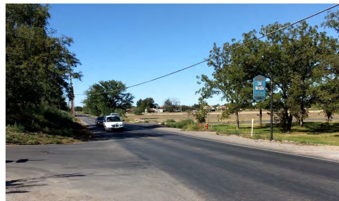
Figure 4.4.1 University Avenue and Bowman Street
