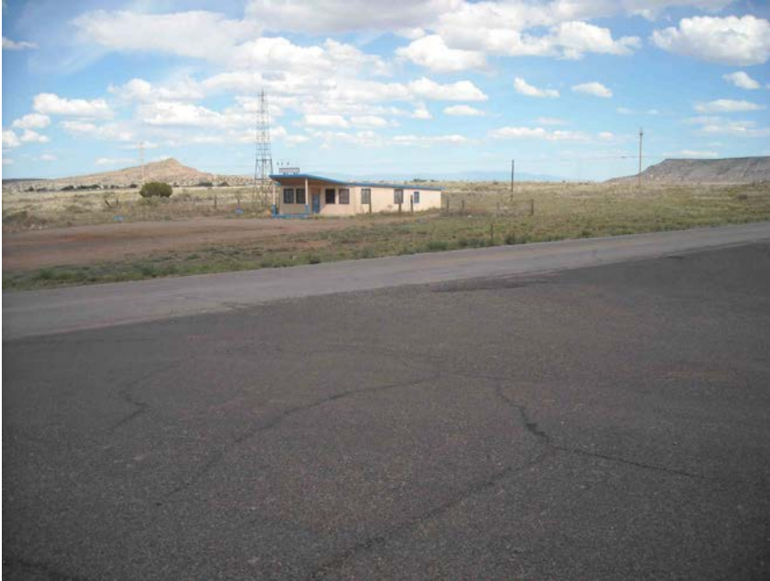
Figure 5 Abandoned building on southeast corner of C084/NM 6 intersection
