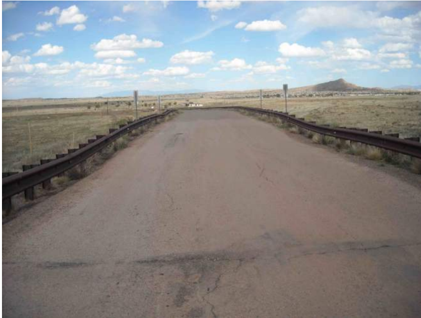
Figure 22. Looking east from top of C084 Bridge
