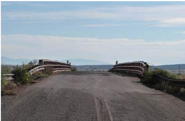
1. Embankment Failure
