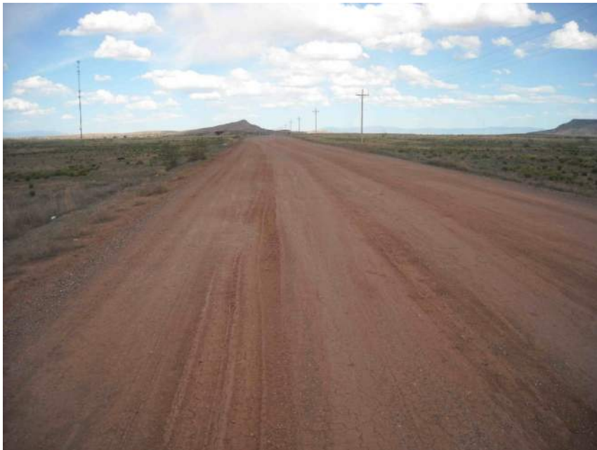
Figure 23. Looking east along C084 from west end of project area
