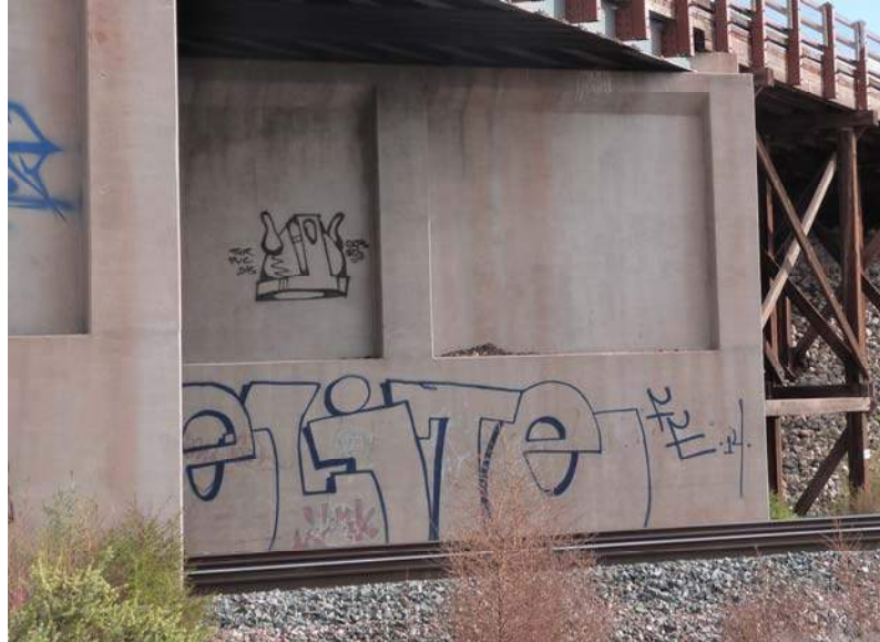
Pier Concrete Walls
