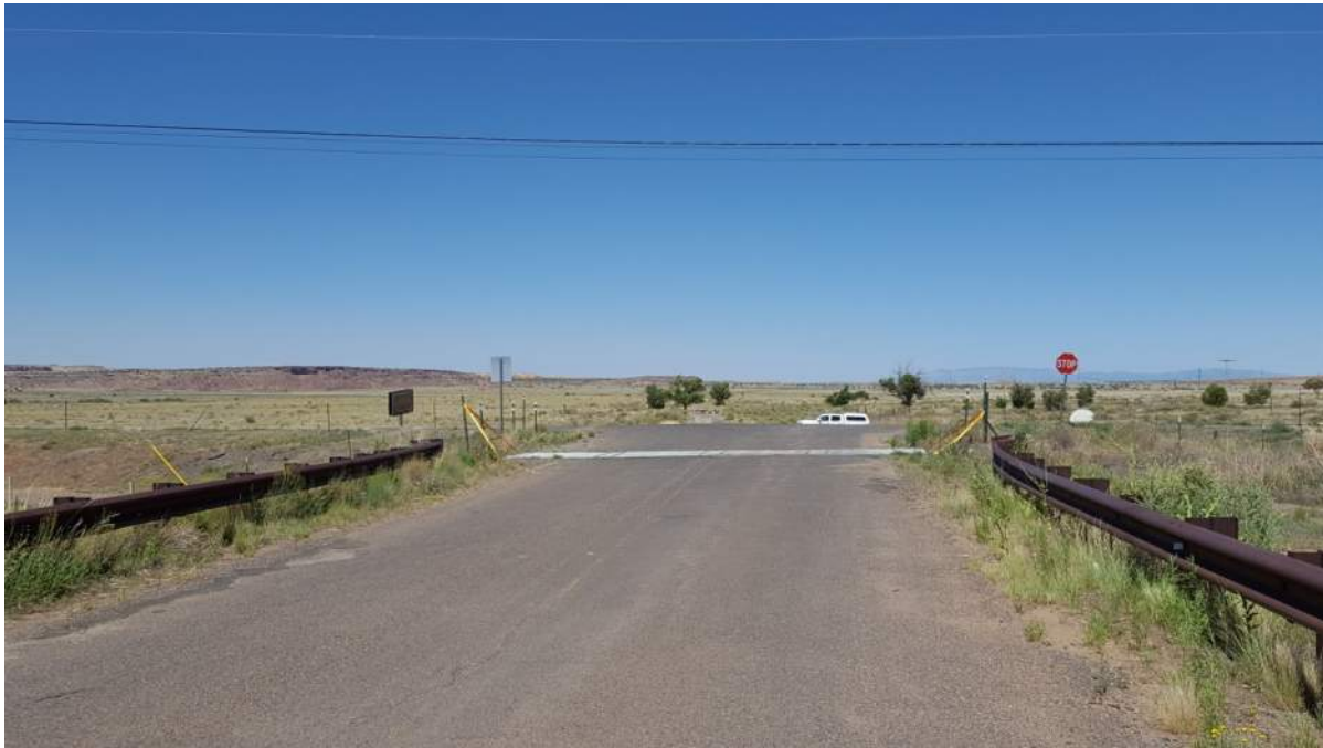
Figure II.A.4 C084 Facing East Approximately 100 feet west of NM 6
