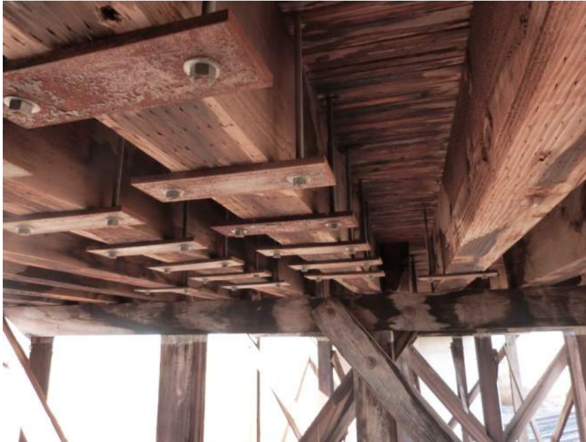
Figure 13. Girders with Straps and Cradles
