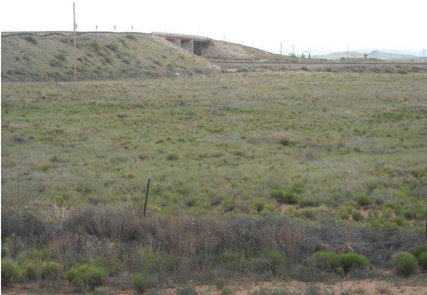
Figure 2 View of C084 bridge from NM 6
