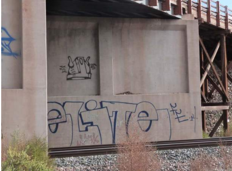
Figure 16. Pier Concrete Walls
