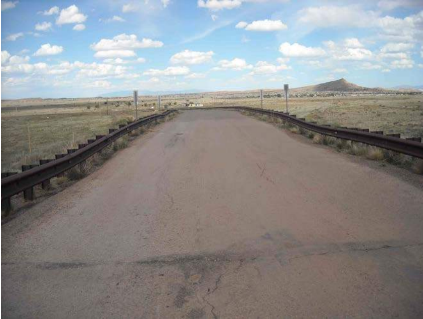
Figure 3 Looking east from top of C084 bridge
