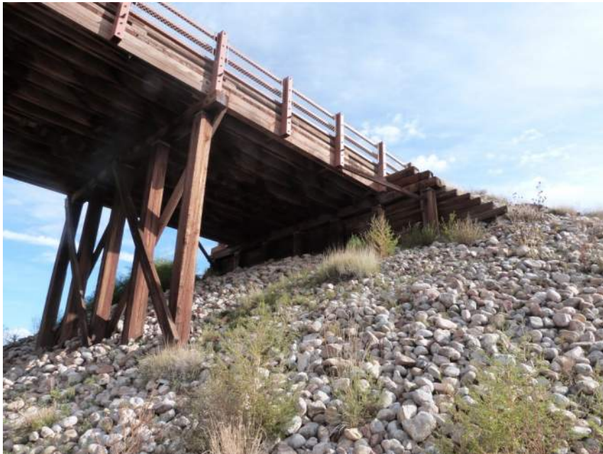
Figure 17. Abutments with Slope faced with Riprap
