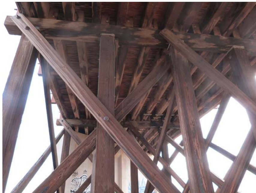
Pier Timber Columns
