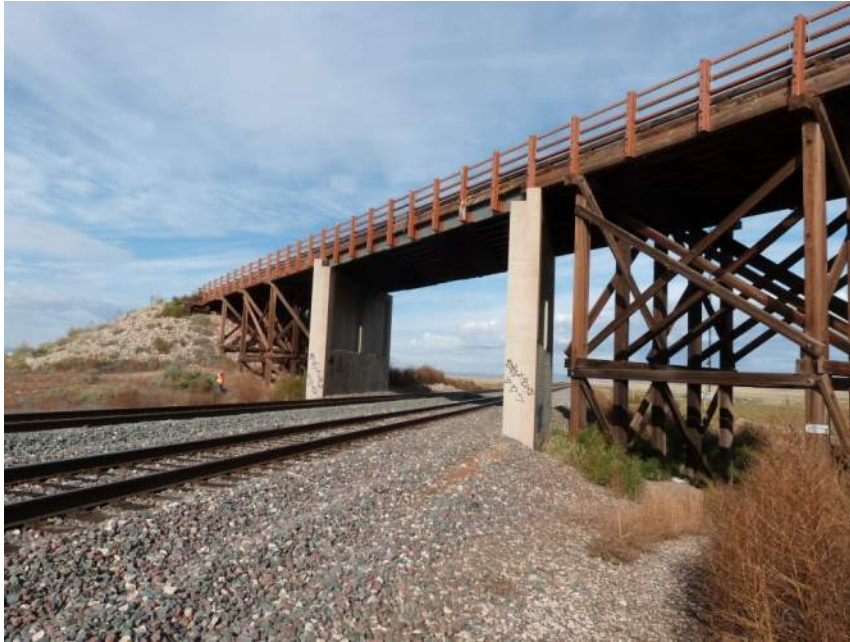
Figure 11. Bridge Elevation View
