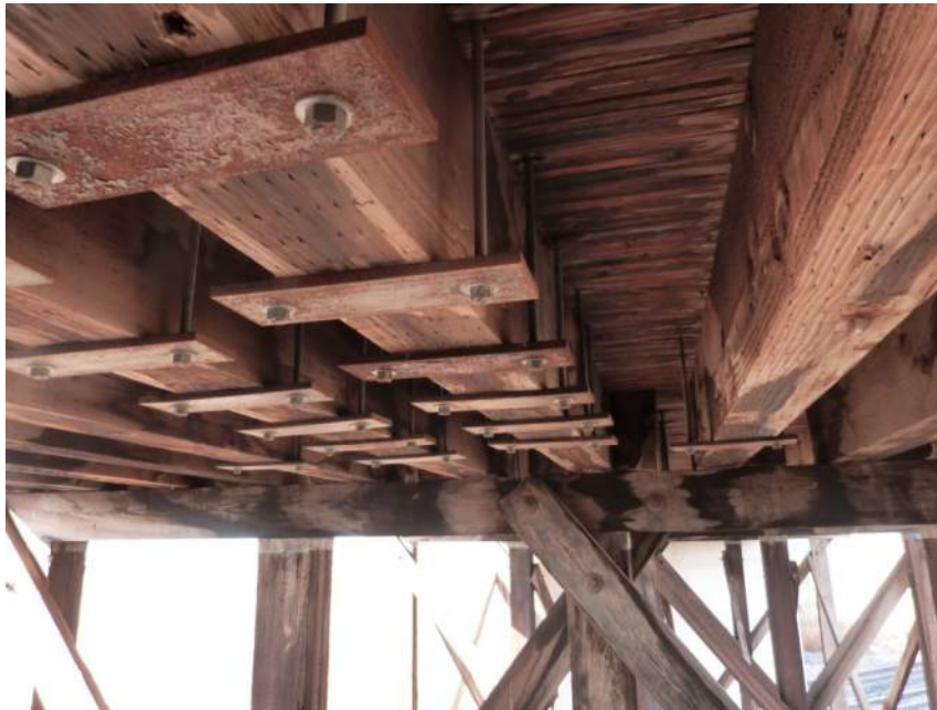
Figure II.A.10 Girders with Straps and Cradles
