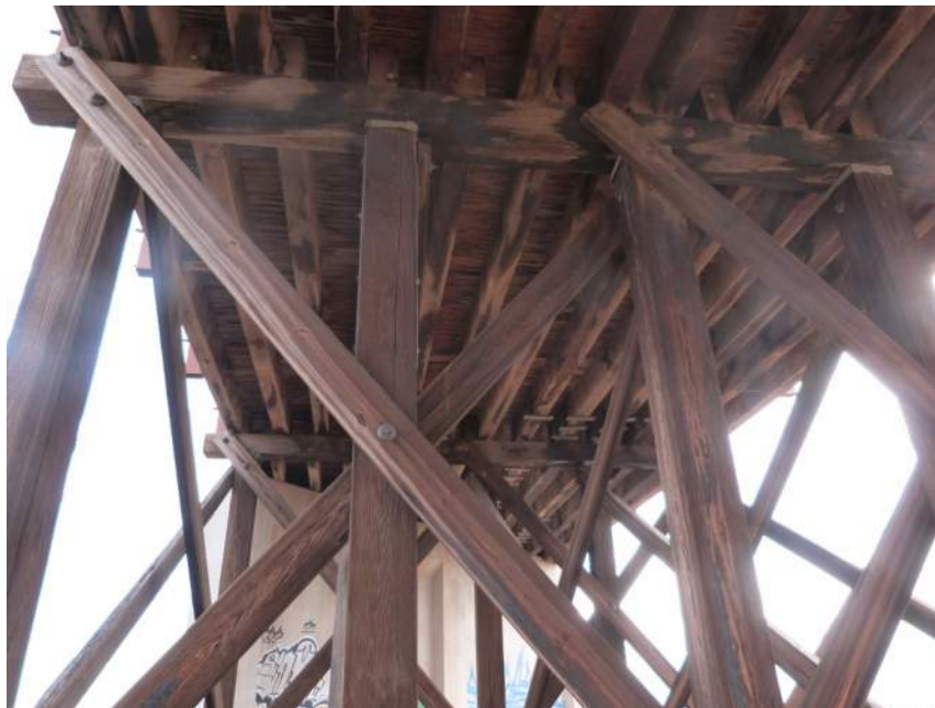
Figure 15. Pier Timber Columns
