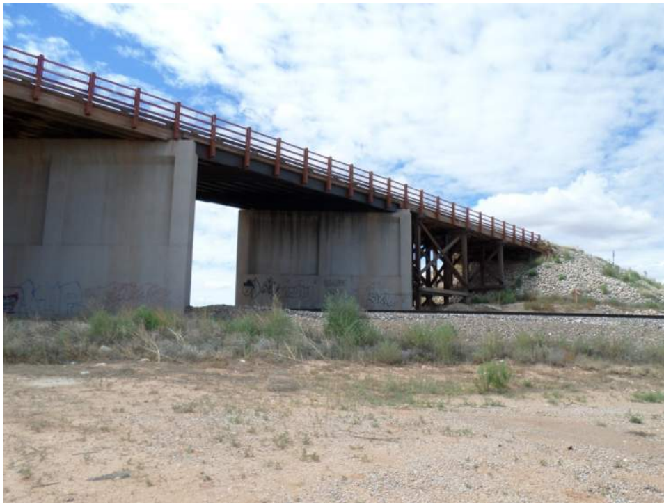
Figure 19. Bridge No. 0002 with Railroad Tracks
