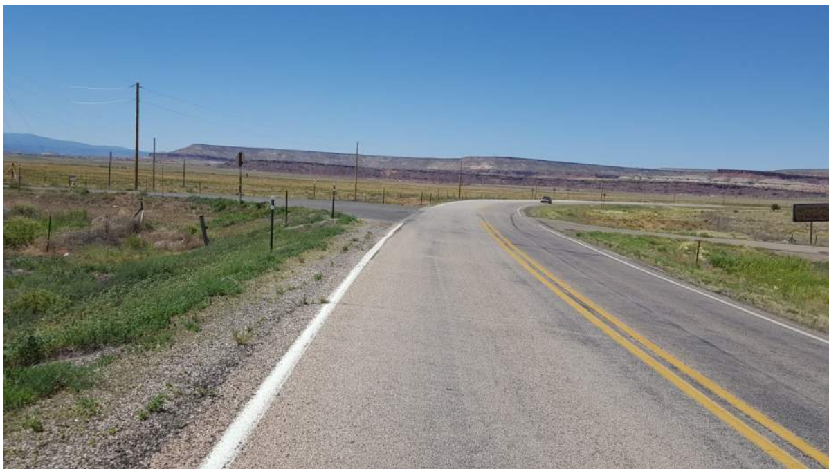
Figure II.A.5 NM 6 Facing North, South of C084
