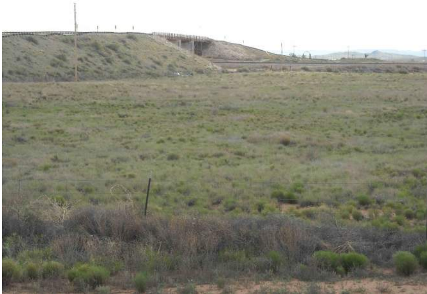
Figure 21. View of C084 Bridge from NM 6
