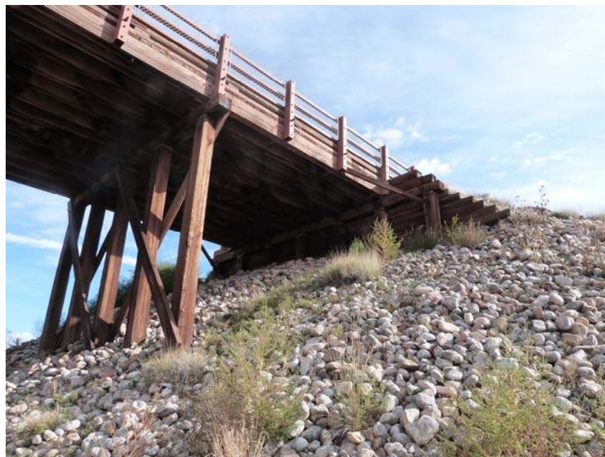
Abutments with Slope faced with Riprap
