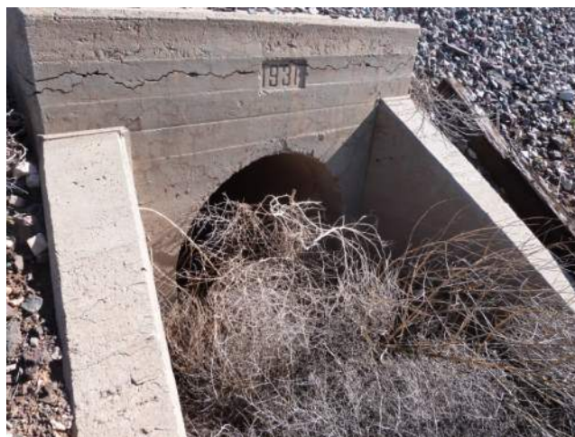
Figure 4: Existing BNSF Culvert
