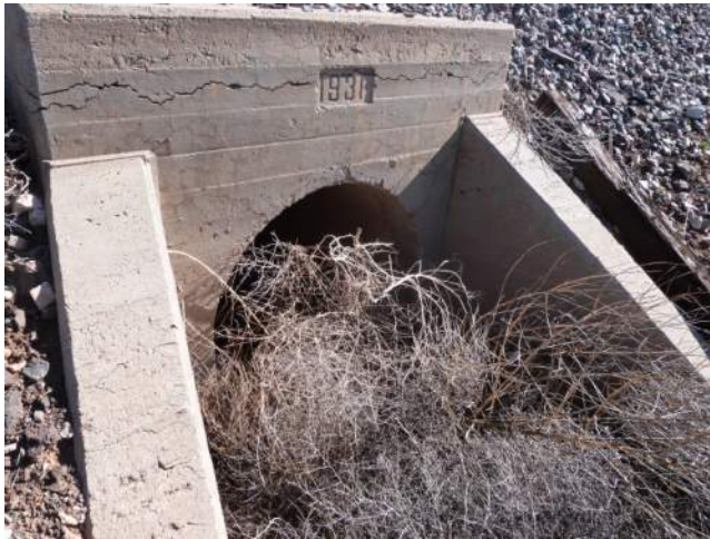
Figure 9. Existing BNSF Cross Culvert
