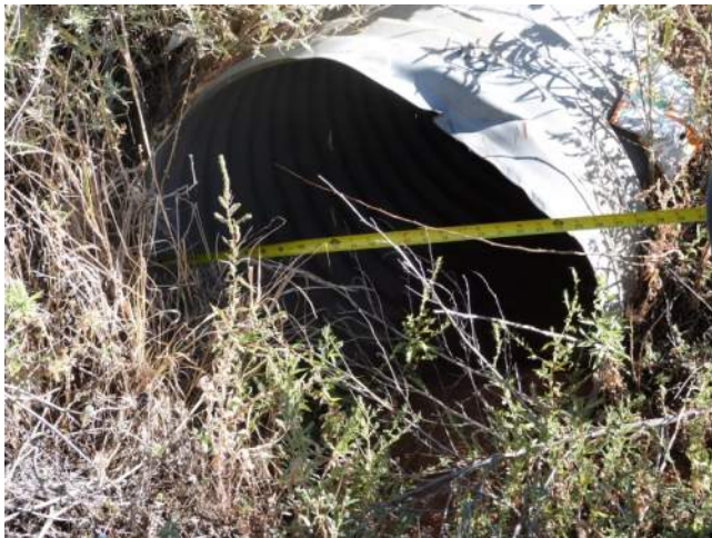
Figure 8. Existing Cross Culverts at NM 6
