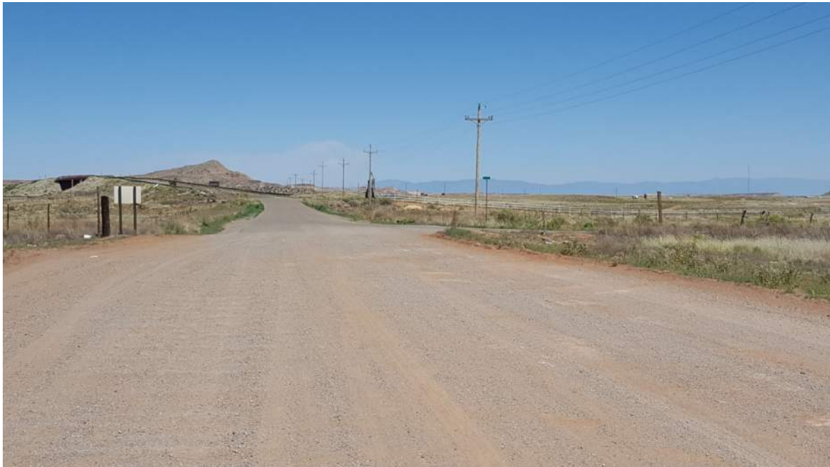
Figure II.A.3 Eastbound C084 near Highland Boulevard, Bridge #2 in Background
