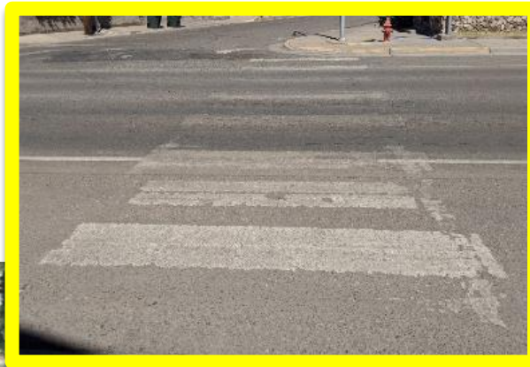
Figure 56: Existing conditions of crosswalk markings, N. Broadway St.
