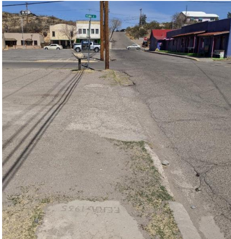
Figure 64: Existing conditions of pedestrian infrastructure in downtown T or C on city owned streets.
