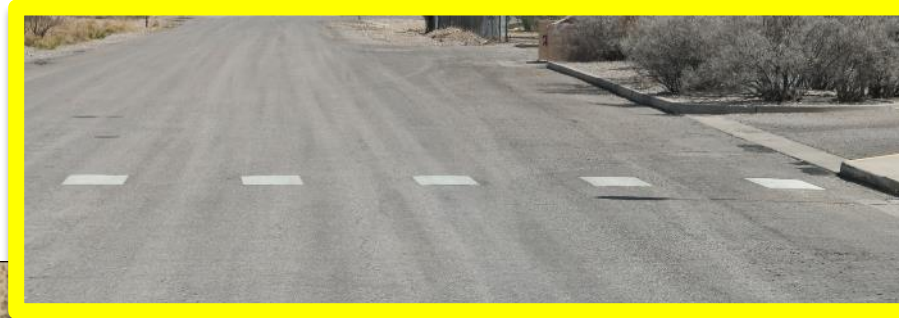
Figure 72: Existing conditions of crosswalk markings, Smith Ave.
