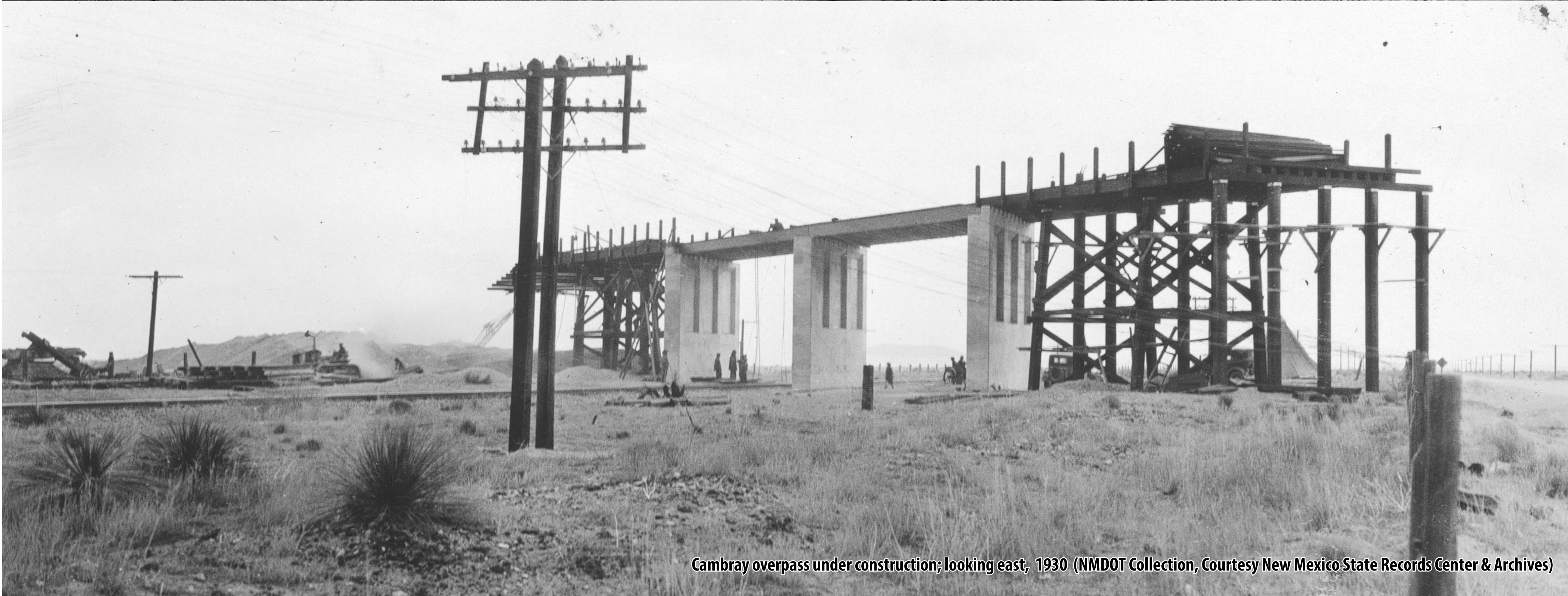
Concrete pier, east approach of Cambray overpass under construction, 1930 (NMDOT Collection, Courtesy New Mexico State Records Center & Archives)
